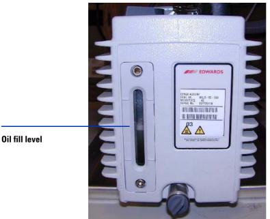
Figure 76 Fluid level window on the rough pump
